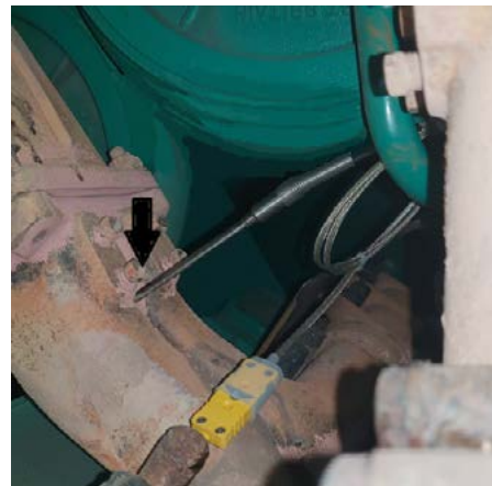
FIGURE 17 INSERT COMPRESSION FITTING WITH SENSOR INTO BUNG
