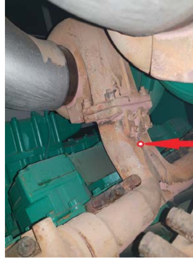
FIGURE 14 MARK WELD-IN BUNG PLACEMENT
